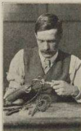
WIRING OF ELECTRIC LIGHT FITTINGS.
