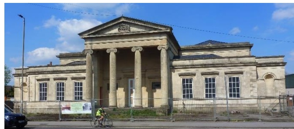
The Devizes Assize Court building in 2022
